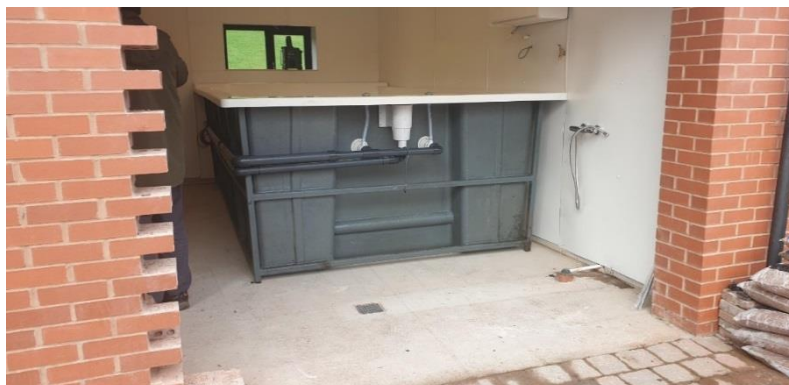
Derwent positioned in building ready for installation
