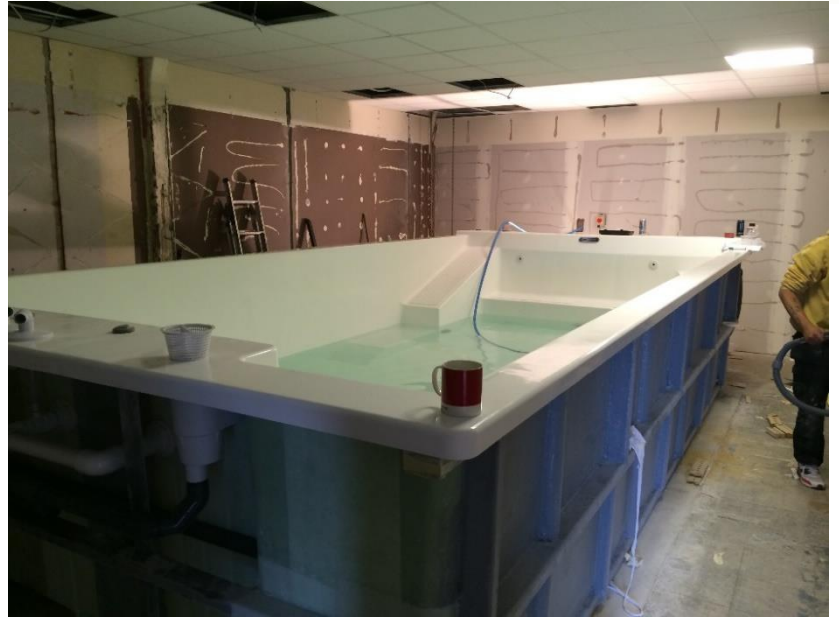
Derwent being filled during installation
