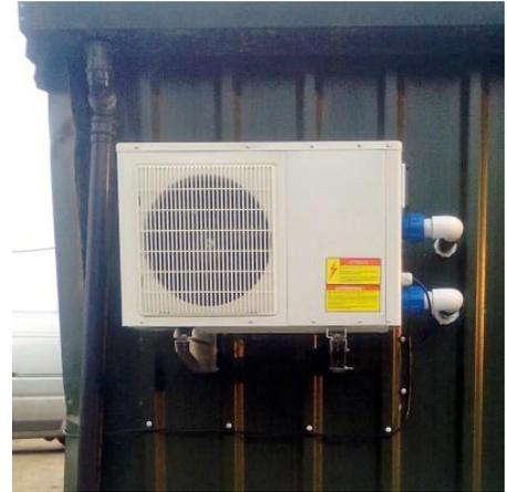
NB. When the ASHP is fitted to the pool plant system, the Balboa heater is used as a backup or as a top up during extreme weather conditions that occasionally occur in the depths of winter.
